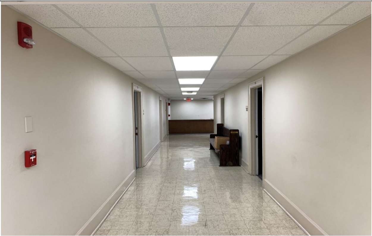
Typical Office Space – 2 nd Floor
