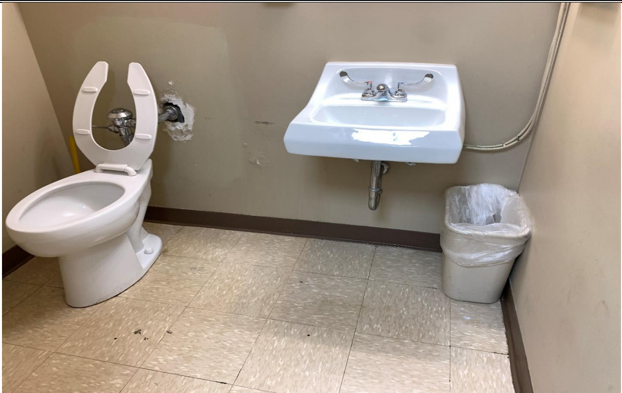
Typical Office Space – 1 st Floor
