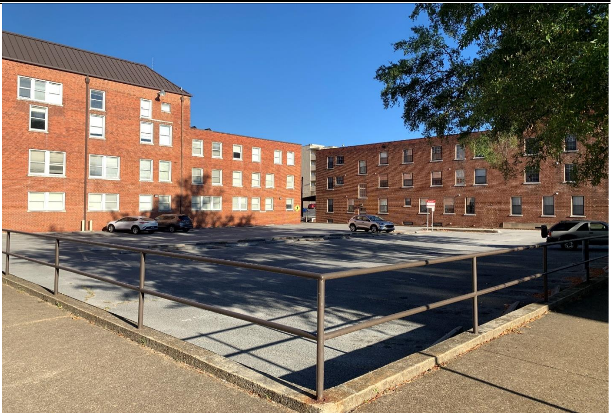
Subject Surface Parking Lot
